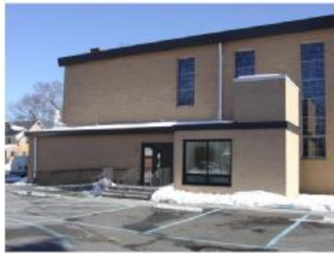
ST. JOSEPH'S ELEVATOR ADDITION
